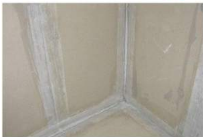
輕隔間角隅補強
