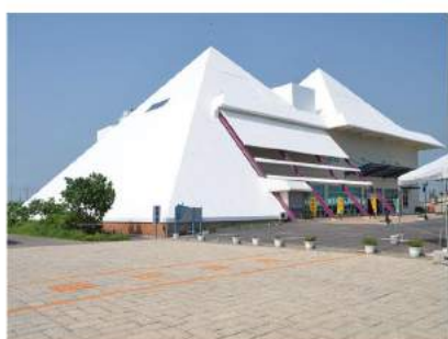
露出防水工法抗UV面塗
