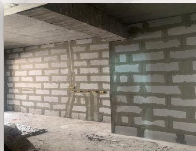
縫隙管線修補
